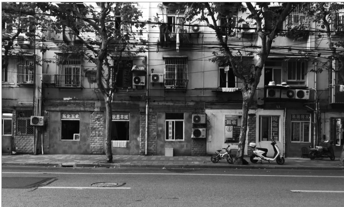
Figure 3. The illegal shops were sealed up with brick walls and restored to windows with temporary advertisement on it. Photo by the author, 2019.
