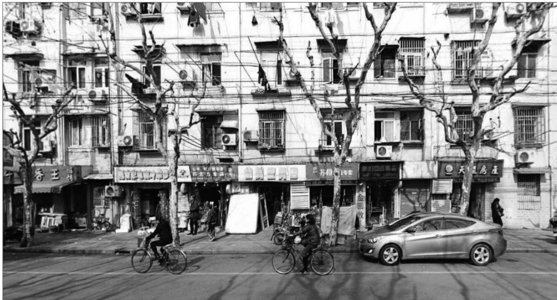
Figure 2. The once vibrant streets shaped by the illegal ground-floor shops in Shanghai. Photo from Baidu maps, 2013.
